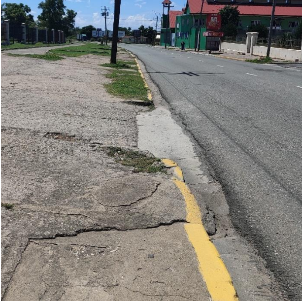
Figure 4-16: Kerb Drain along perimeter of compound
