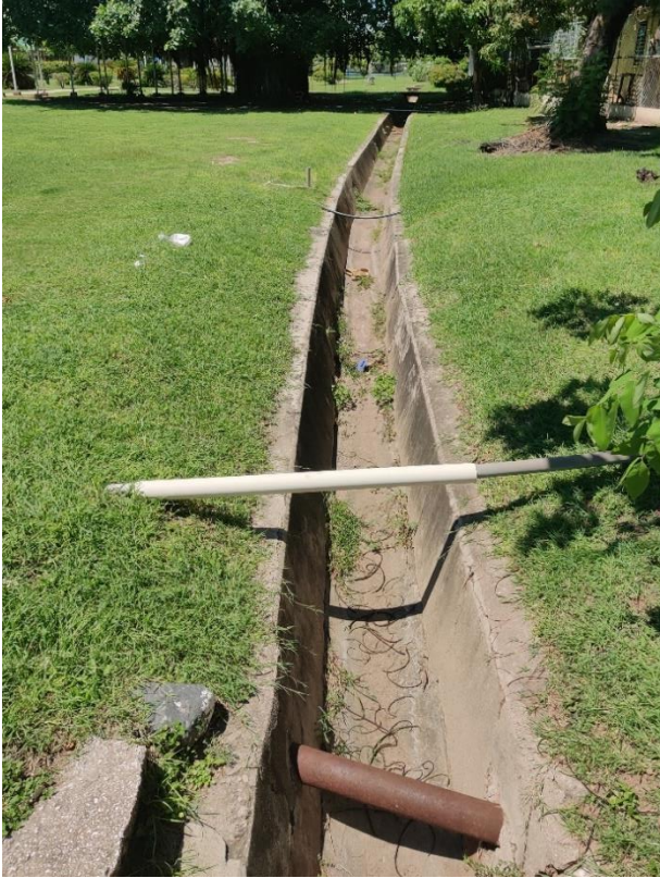
Figure 4-15: Existing Heroes Circle internal drain (uncovered)
