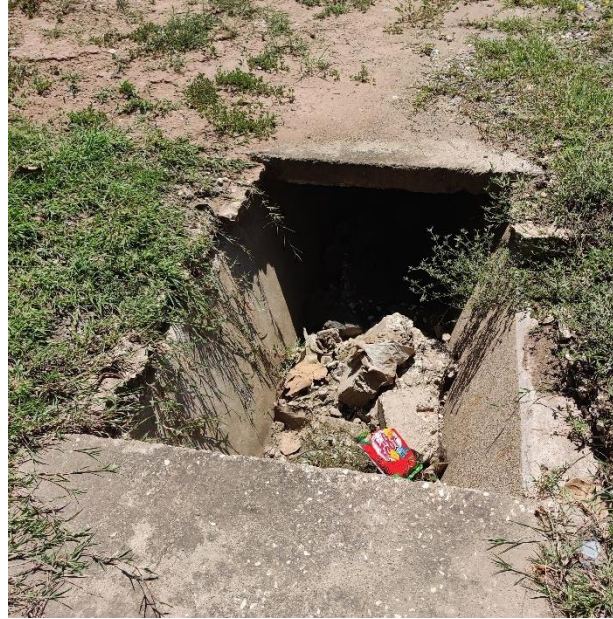
Figure 4-17: Existing Heroes Circle internal drain (covered)
