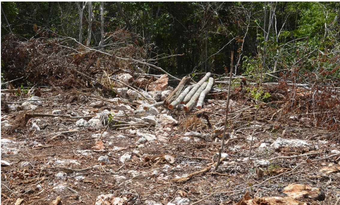
Figure 4-29: Posts cut and stored along clearances.
