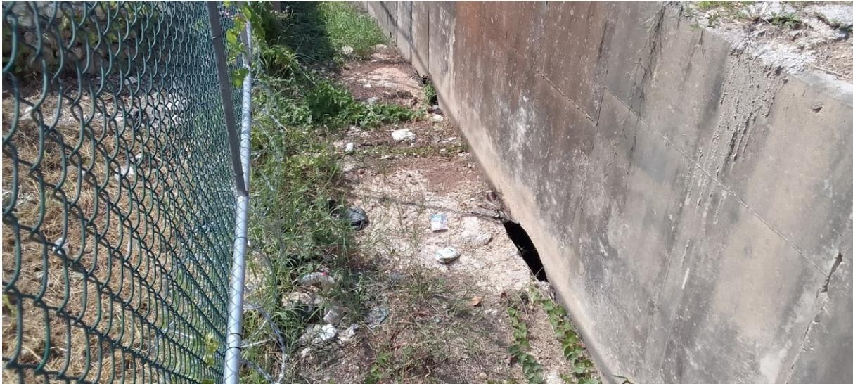
Figure 4-33: Concrete water channel north of the waterwheel – drains seen at base of wall (Conolley photo 2022.)
