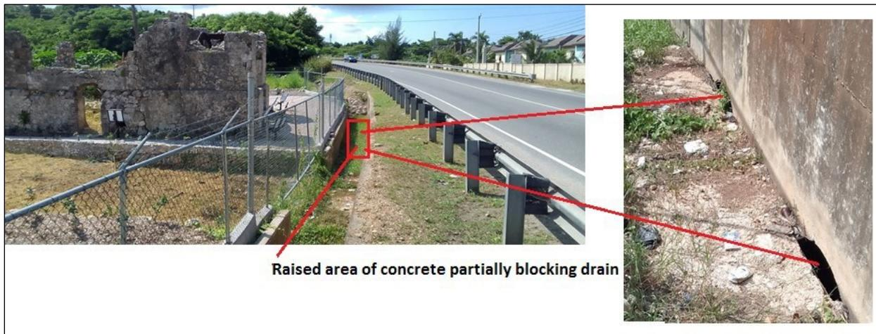
Figure 4-34: Water Channel drainage 1 (Adapted area in Red by Conolley and associated text by Conolley. Conolley photo 2022.)
